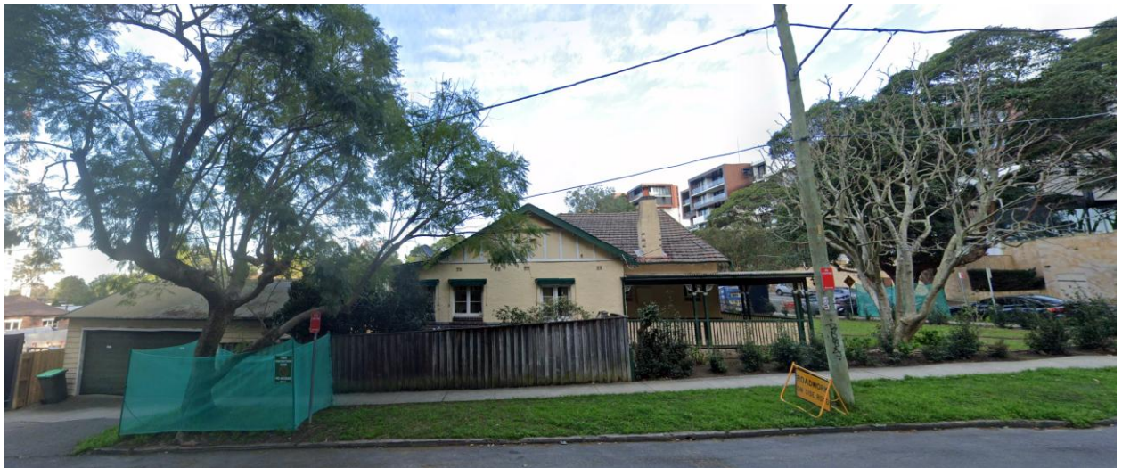
Figure 6 Subject site as viewed from Canberra Avenue.
